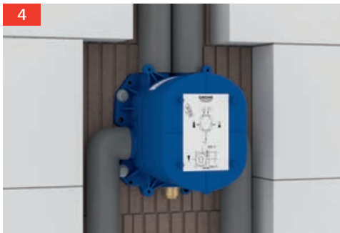
4 Make good wall recess Note markings indicating the correct installation depth
