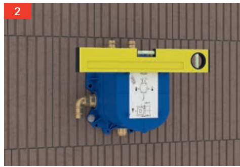
2 Align the concealed valve Mark drill holes, drill holes and install fitting box
